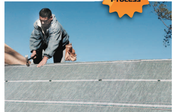
The ALCO Shield 15 Synthetic underlayment product offers installers ease of installation because of weight, roll width and its non-slip properties. The unique stitched pattern provides strength not found in felt paper.
